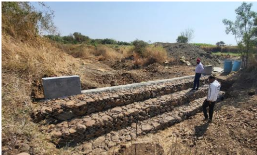
Gabion with core wall at Bitargaon
