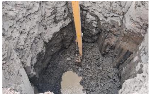
Village Kamone Community Irrigation Well Work 50 Feet done
