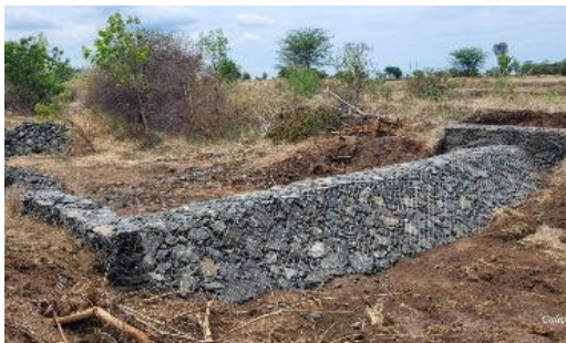
Gabion structure at Aljapur
