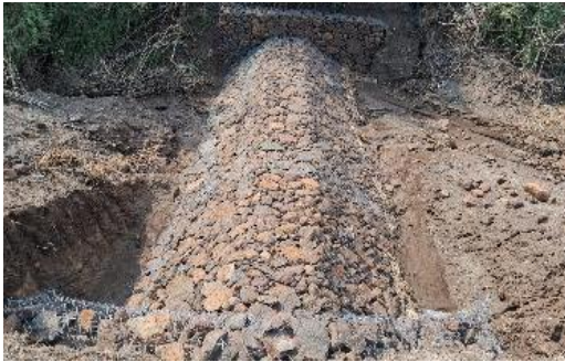
Gabion structure at Balewadi
