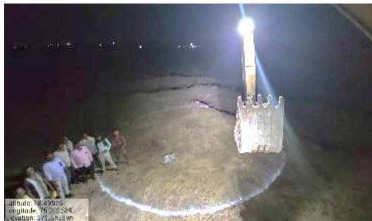
Village Kamone Community Irrigation Well Mark Out
