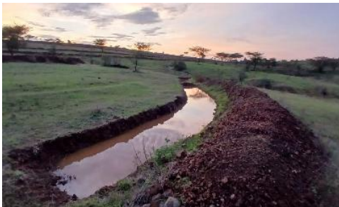
Deep CCT at Kamone
