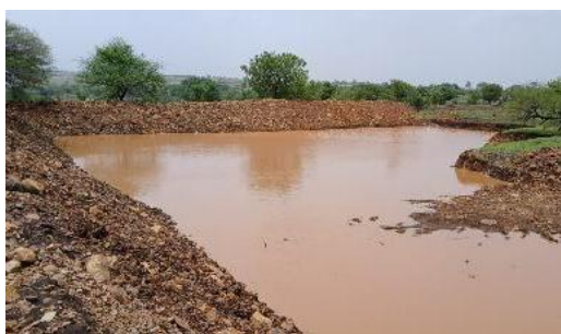
Waterbody Restoration Hirya Mal Work At Balewadi Work Completed
