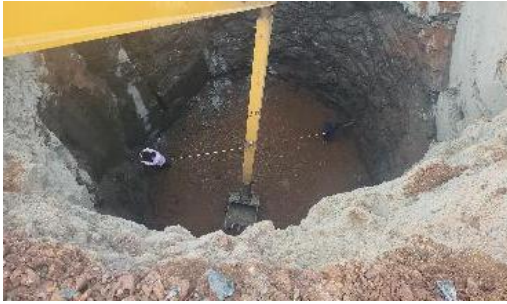
Well measurement after completion of work
