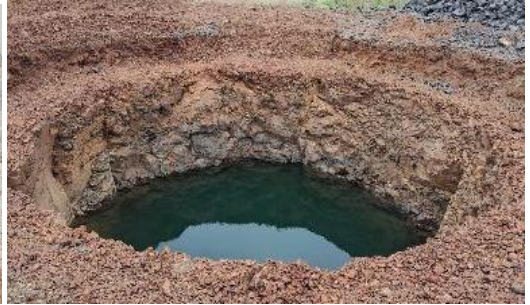
Village Kamone Community Irrigation Well Work 50 Feet work done
