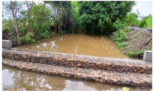
Gabion with core wall at Bitargaon
