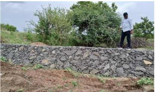
Gabion structure at Aljapur
