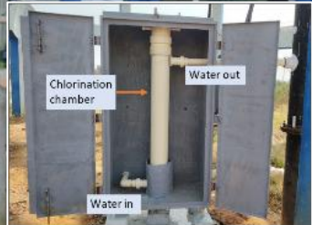
Automatic Chlorination & Online Monitoring System – an innovative, patented solution for ensuring water safety and service reliability.
