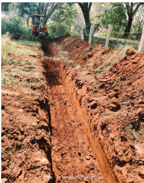
Water Absorption Trenches
