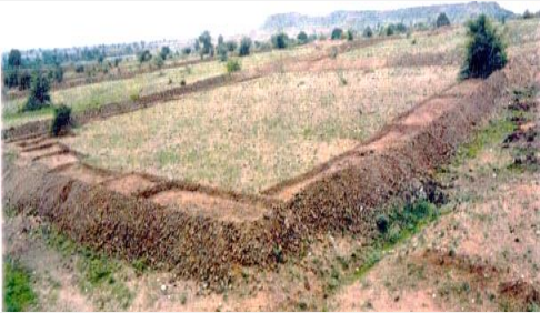
Repair Farm Bunds, Haryana
