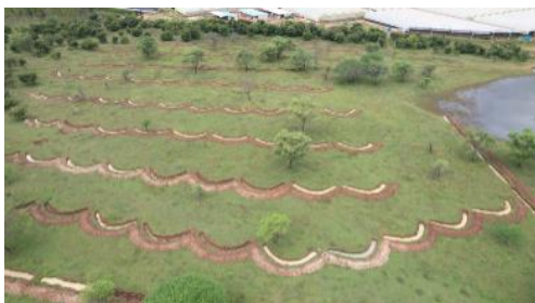
Continuous Contour Trenches
